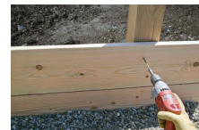
Exterior timber element fastening
