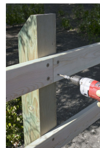
Railing fastening
