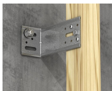
Connect timber battens.
