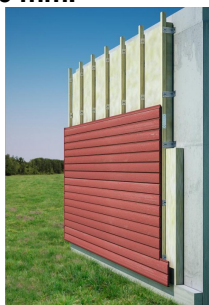
Cladding installation
