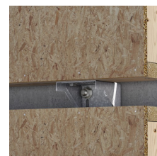
Brackets set below, on slab edge
