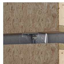
Brackets set below, on slab edge
