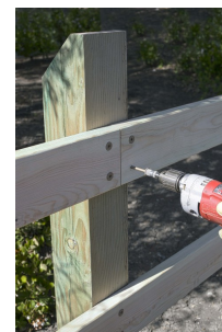
Railing fastening
