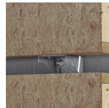
Brackets set below, on slab edge
